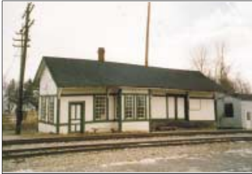
Photo 1. The foundation of the depot is sinking, necessitating repairs. Moving the depot to a new foundation may actually make rehabilitation easier.
